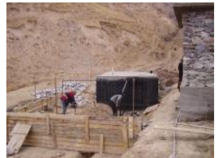
Construction of reservoir, Dashti Maidon Village
